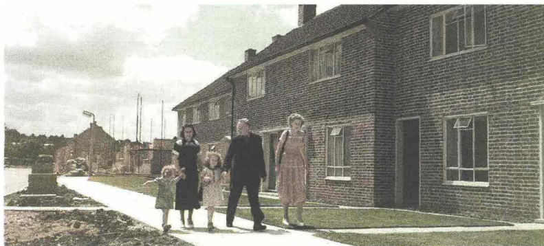
CRAWLEY, NEW TOWN
